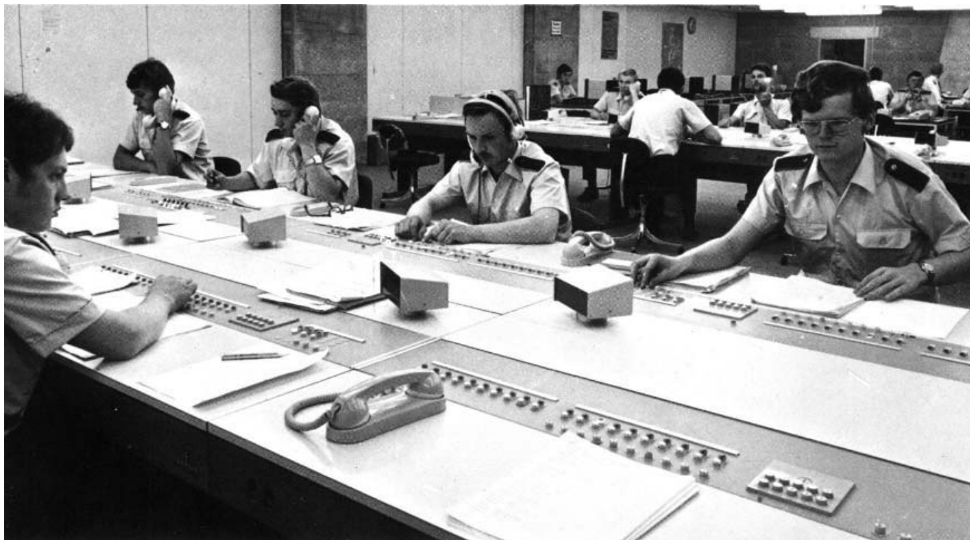
The large telephone exchange in Olympic Stadium (20 operators for ca. 2,000 extensions, 390 trunk lines, 186 cross connections to the sub-exchanges)
